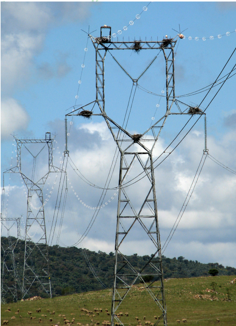
Transmission line tower equipped with bird-saving devices
