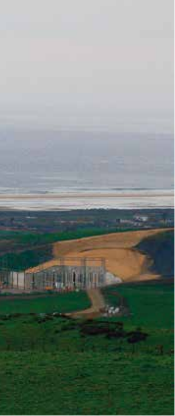
Tarifa station for the Spain-Morocco interconnection. / REE
