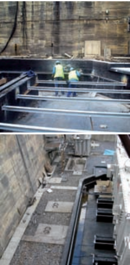
Containment systems. SE Gueñes.
