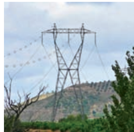
Installation of bird flight diverters. Laguardía-Logroño.
