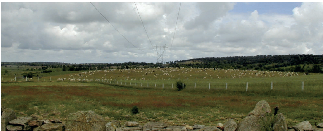
L/220 kV Villalcampo-Villamayor.
