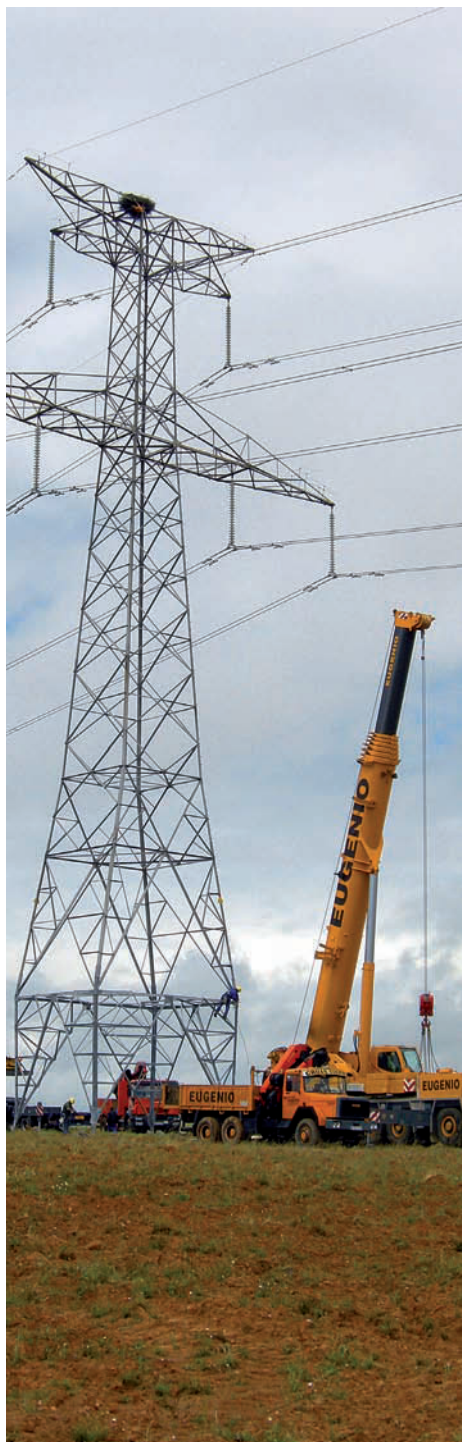
400 kV Line José María Oriñ-Arañuelo. Works on facilities without removal of nest.
