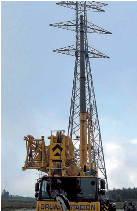
Hoisting of tower with crane.
