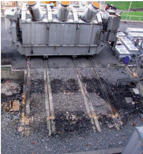
Fitting of oil collection pits in power machine.
