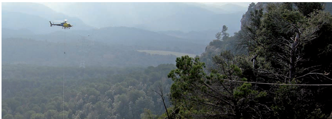
400 kV Line Setmenat-Vic-Bercarnó. Hanging of cable by helicopter
