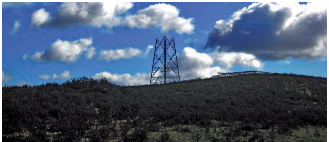
220 kV Line under construction. Puebla de Guzman.
