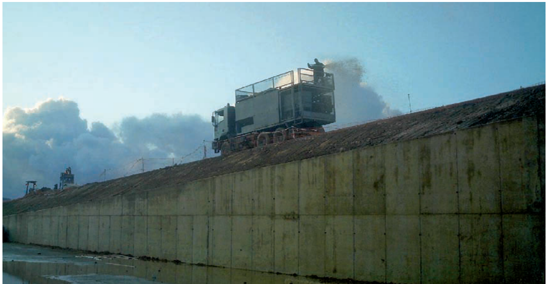
Hydro-sowing Pesoz Substation.
