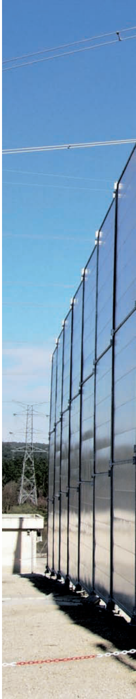
Installation of acoustic screens
