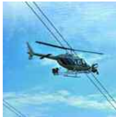
Installing of bird-protection under voltage
