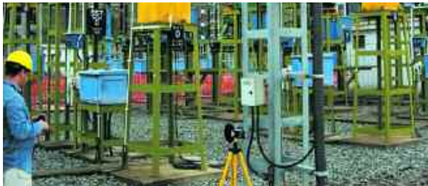
Measuring of electromagnetic fields and noise
