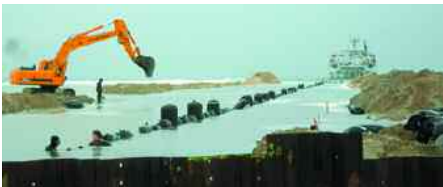
Laying of the second Spain-Morocco interconnection cable in the Estrecho Nature Reserve
