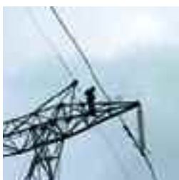
Installation of devices to discouraging nesting on the Sanabria-Mudarra Line.
