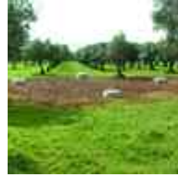
Tower foot during construction of Balboa-Portuguese Frontier Line, showing restoration of the affected ground.
