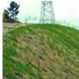
Evolution of recovering a slope at the Boimente Substation.
