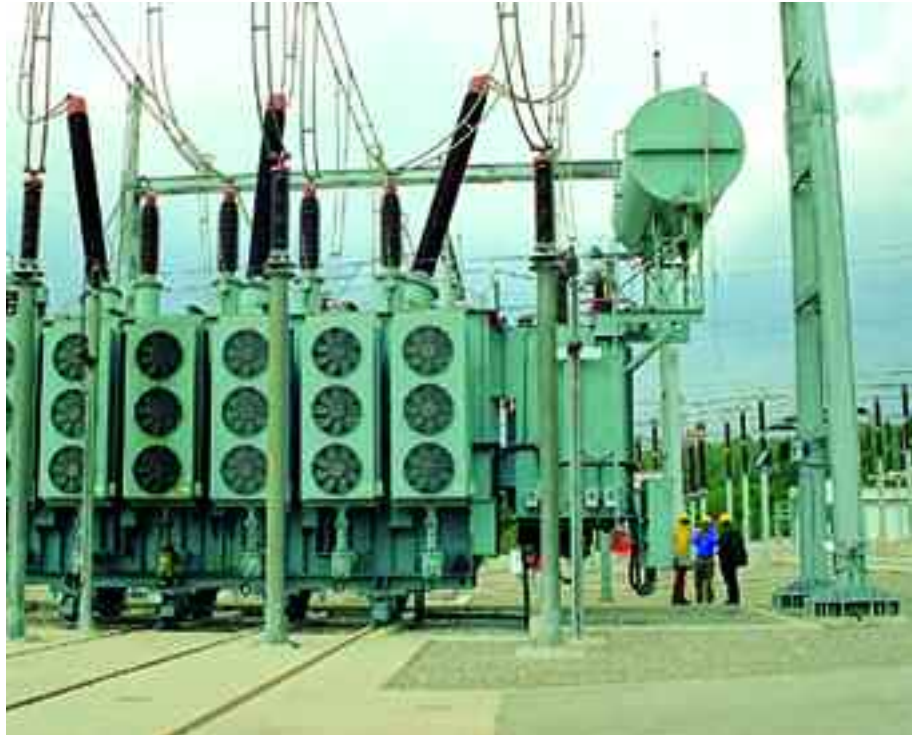
400/110 kV power transformer with collecting oil pit. Calders Substation.
