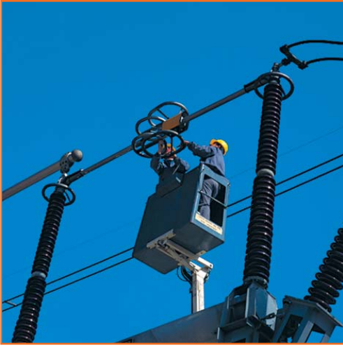
Cleaning the contacts of a switch.
