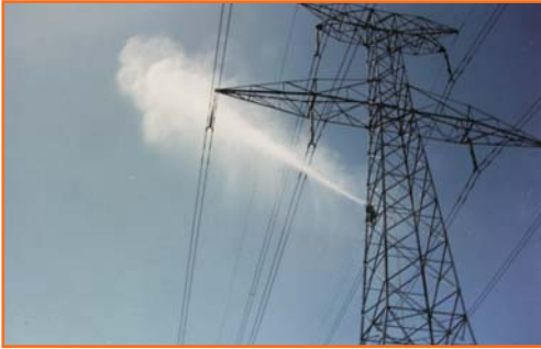
Washing electric glass insulators using trucks.
