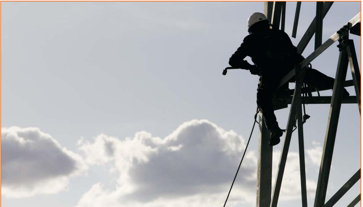
An operator on a tower carrying out maintenance works.
