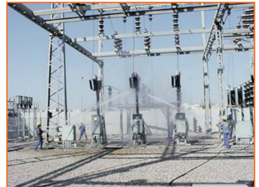
Live working for substation cleaning.
