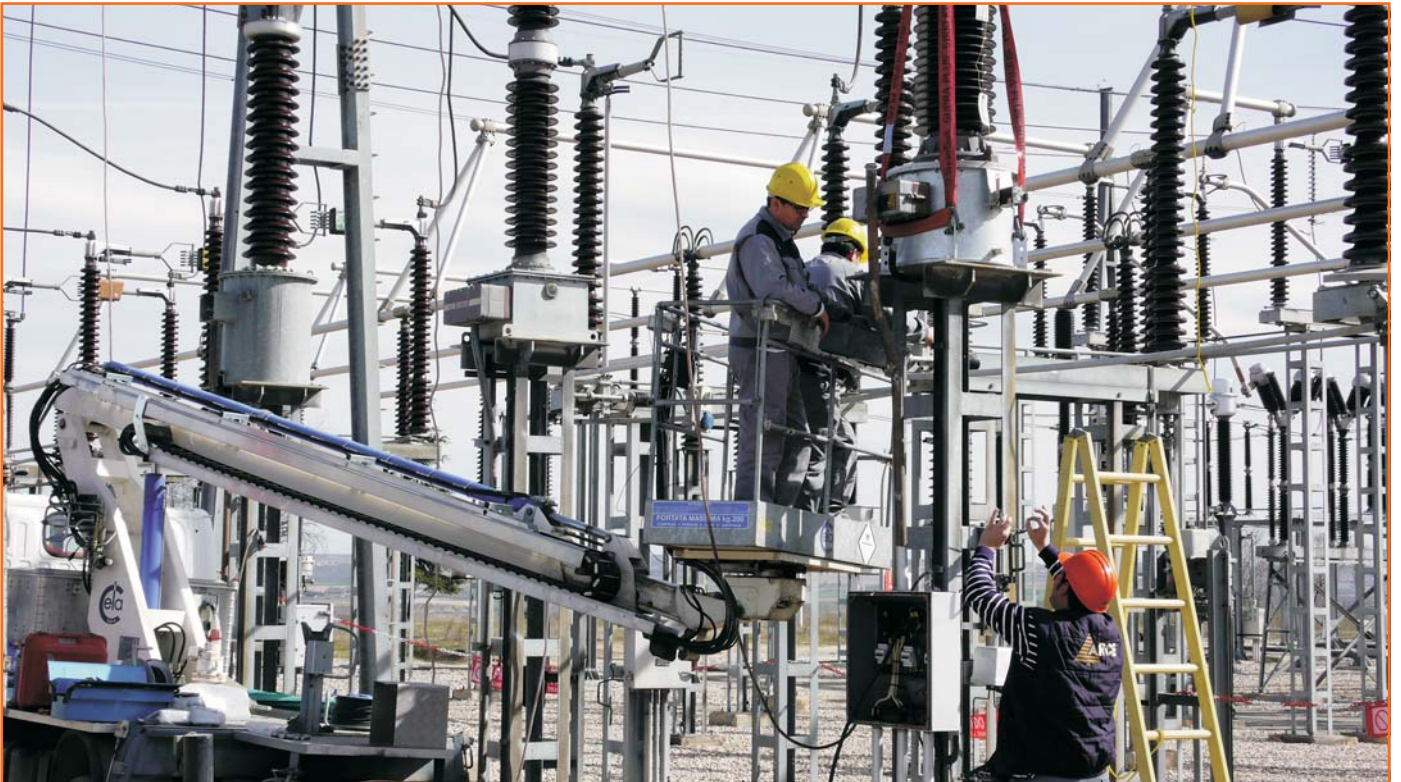
Inspection of a voltage transformer in a substation.
