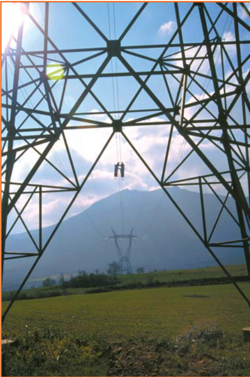
Workers carrying out maintenance.
