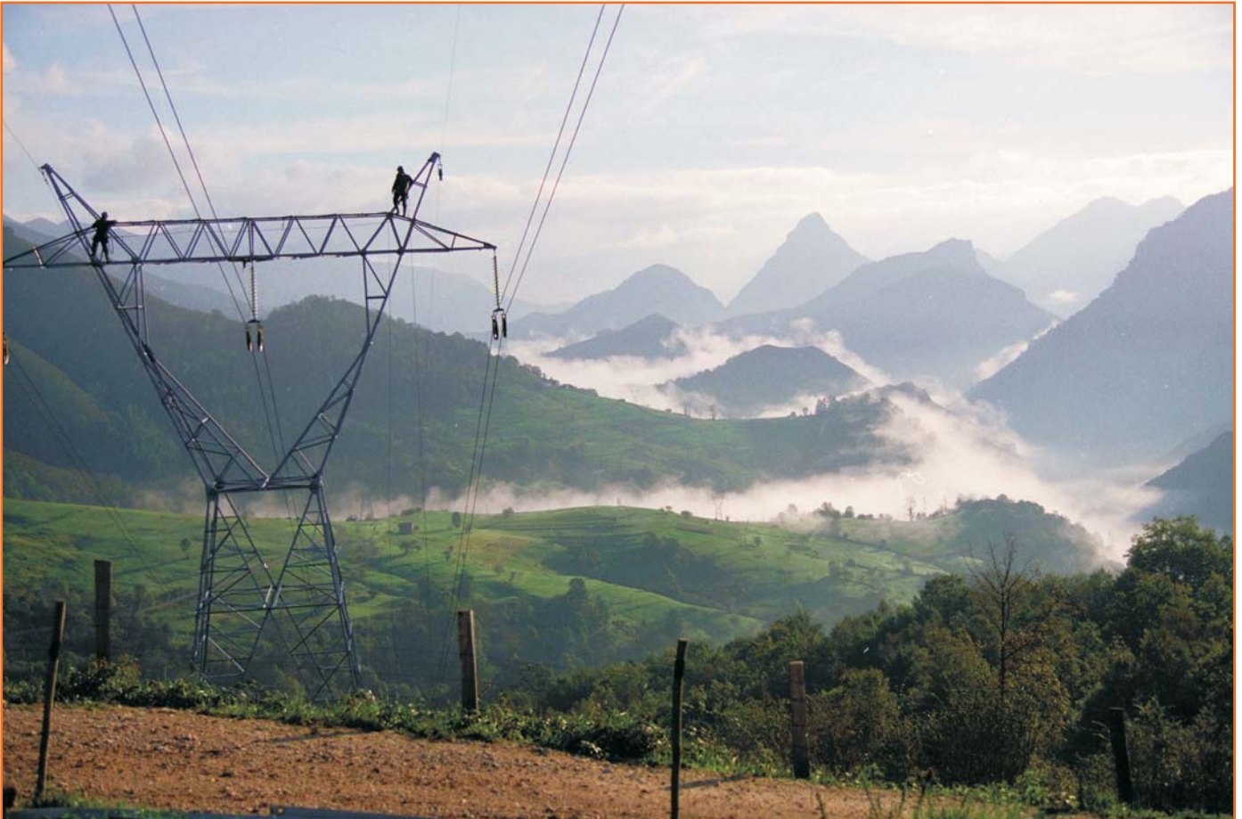
Operators on a tower carrying out maintenance works.
