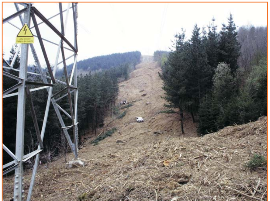
State of a line after the felling and pruning process.
