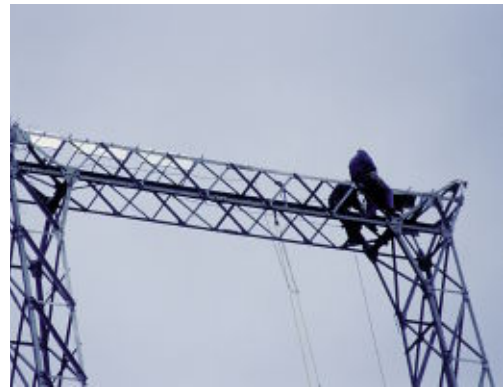
Installing anti-nesting devices
