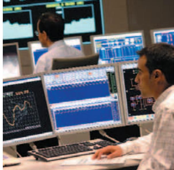
in the grid and generation nodes, as well as consumption, voltage values, etc.). The system processes, also, 25,000 digital variables (circuit breakers and isolator switches position, etc.) and issues the respective remote control instructions for 4,500 variables.
